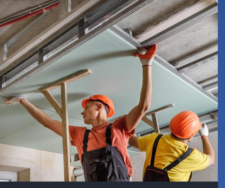
Drywall Installers measure, cut, and fit drywall sheets for installation on walls and ceilings in order to prepare various surfaces for painting and finishing.
